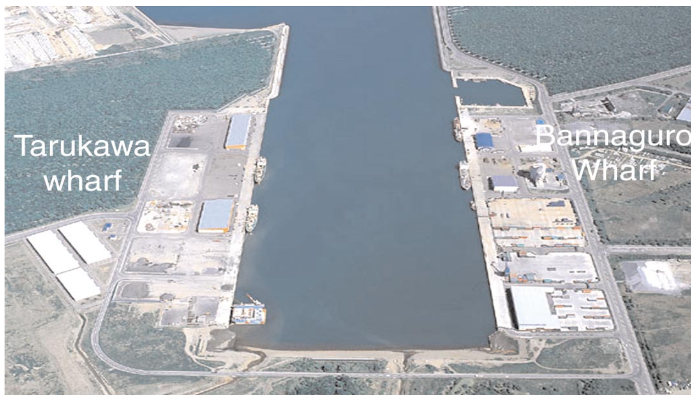
Ishikari Bay New Port—Tarukawa Wharf and Bannaguro Wharf
