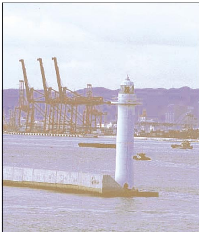
Kobe—No. 7 Breakwater East Light
