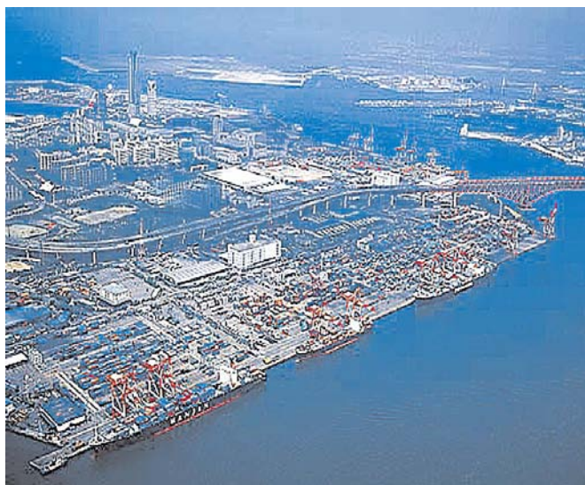
Osaka Ko—East Container Terminal
